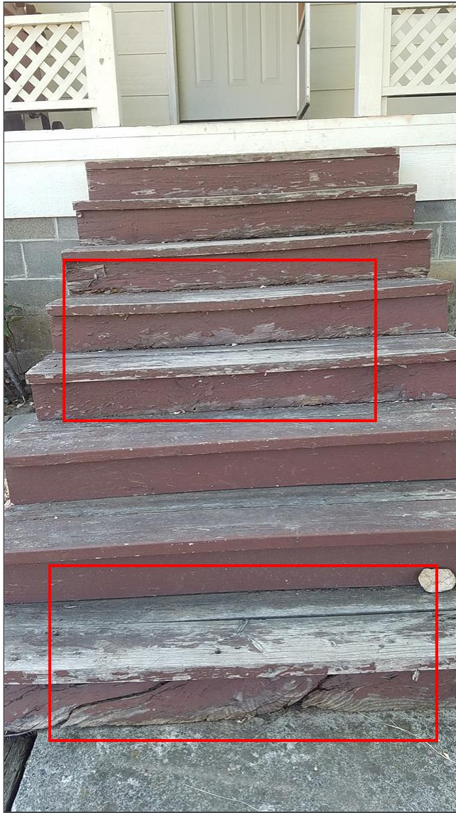
(2) Back steps to upper deck are failing and are a safety hazard. Recommend rebuilding steps properly prior to use.
